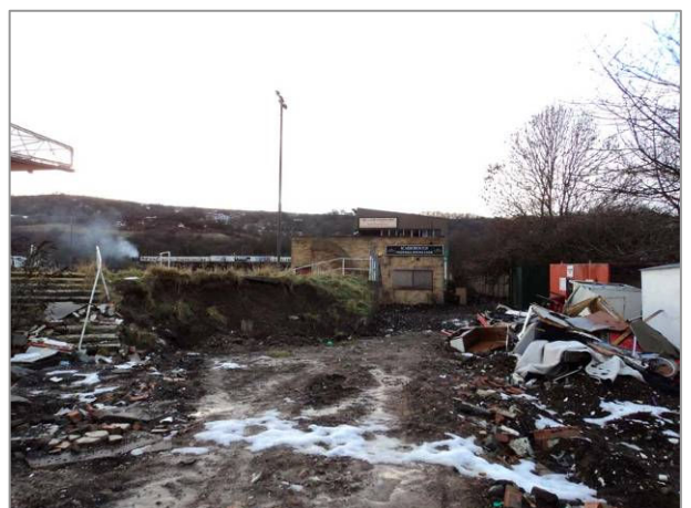
Photo 12: McCain Stadium – Dug up driveway from main entrance
