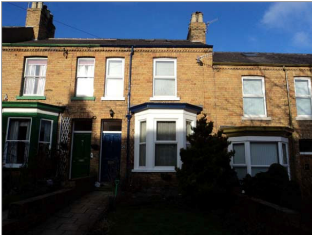
Photo 35: Traditional terraced housing with bay windows and vertical emphasis to the north of the site
