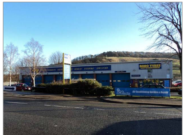
Photo 32: Single storey retail warehouse along Seamer Road
