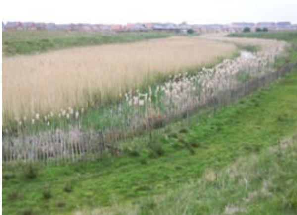
Image 6.9: Example of attenuation pond
