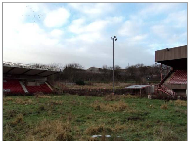
Photo 10: McCain Stadium – Northwest terrace
