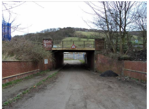
Image 3.8: Height restricted railway bridge
