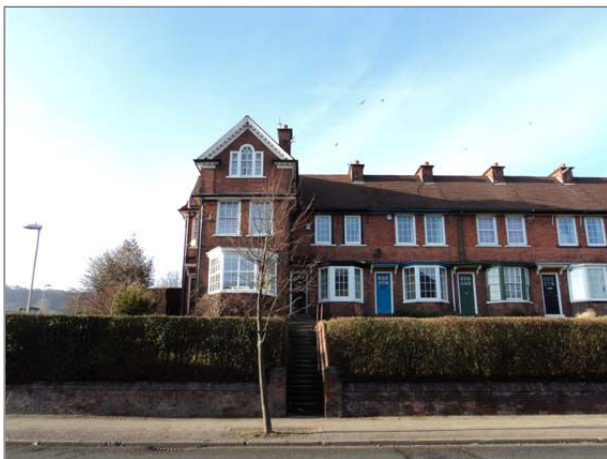
Photo 31: 2-storey residential terrace with end 3 storey house along Seamer Road
