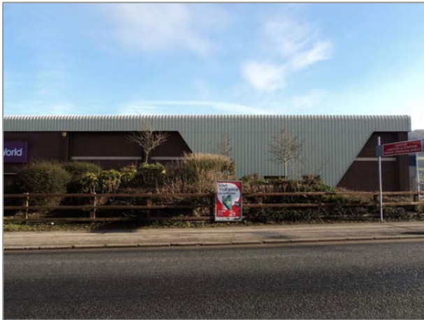
Photo 29: ‘Inactive’ elevation of retail warehouse along Seamer Road
