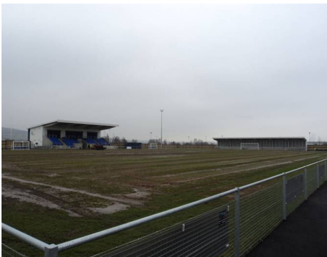
Ground from the northwest corner
