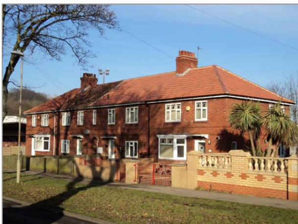
Photo 23: Example of small residential terrace close to the site
